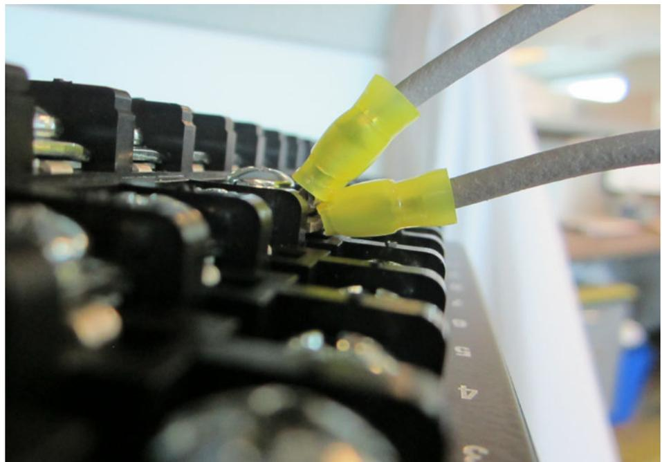
Figure 2-31: INCORRECT INSTALLATION METHOD (lower lug reversed)
